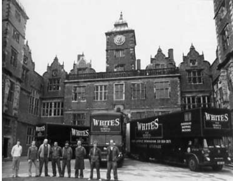
A posed picture showing furniture being removed into store during renovation of the hall in the 1980s
